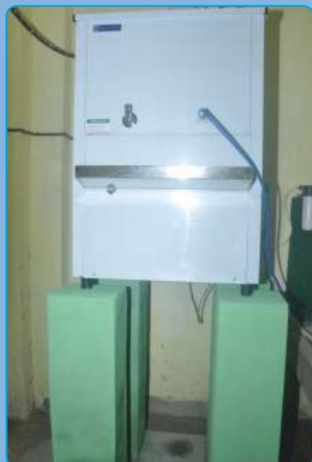
Water Purification Plant
